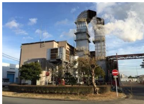
Takasago area facilities
